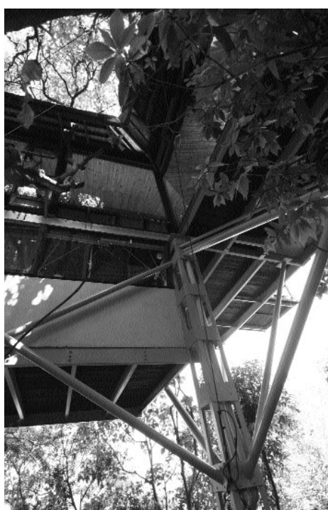
The steel skeleton
